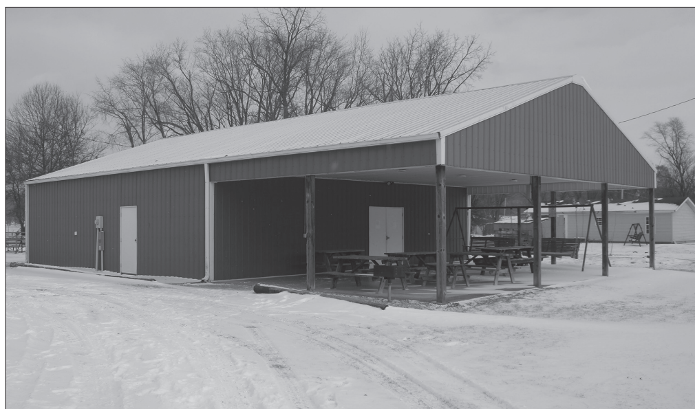
The multi-purpose building in the town park at Paragon is set to become a new Voting Center for this year's elections. (Keith Rhoades photo / MCC)
